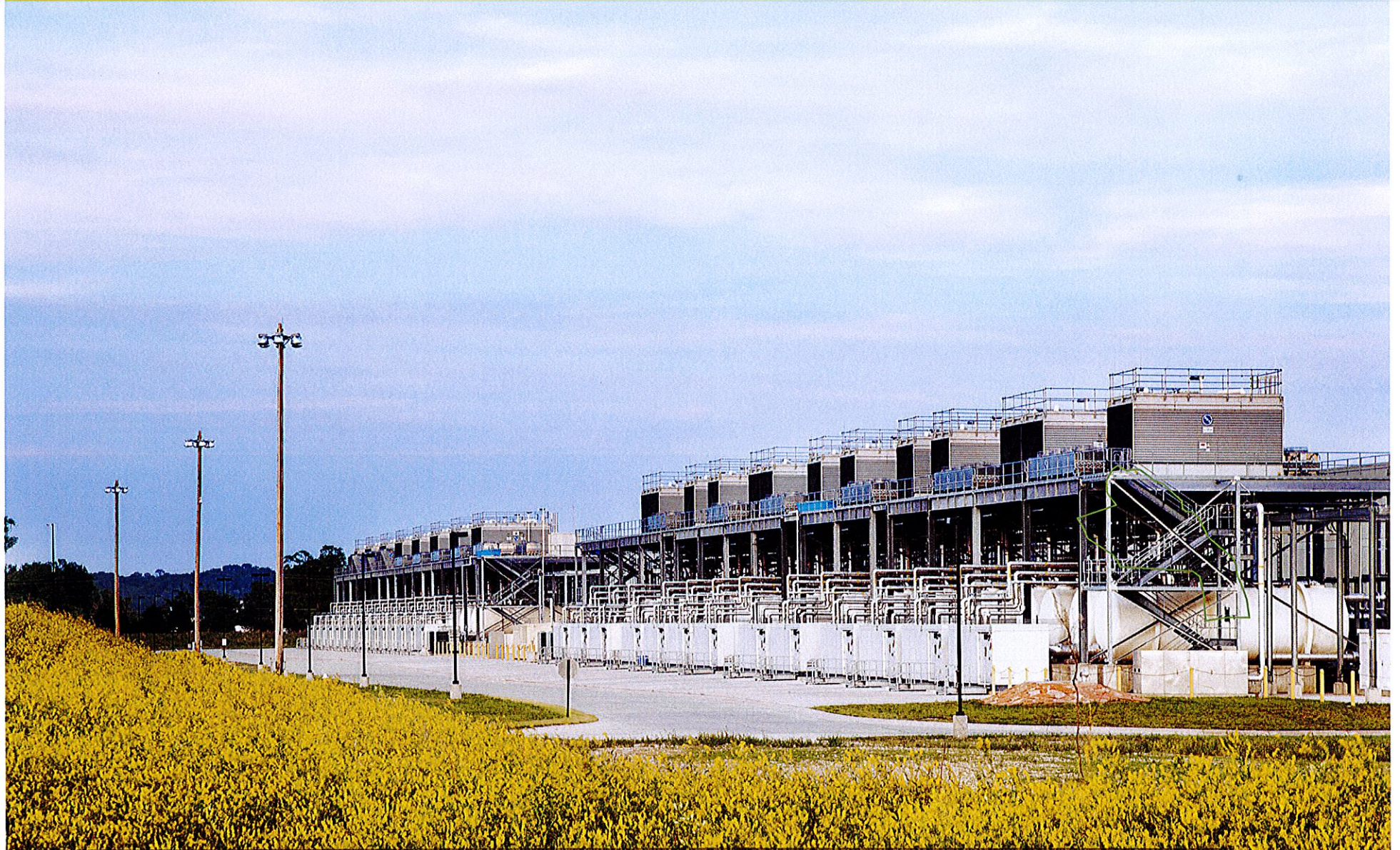
Opportunities for new industry like this Google Data Center, Council Bluffs, Iowa - 130 jobs, 975 acres. (Photo via Google.com/datacenters ); The Dalles, Oregon data center has 80 jobs, 37 acres
